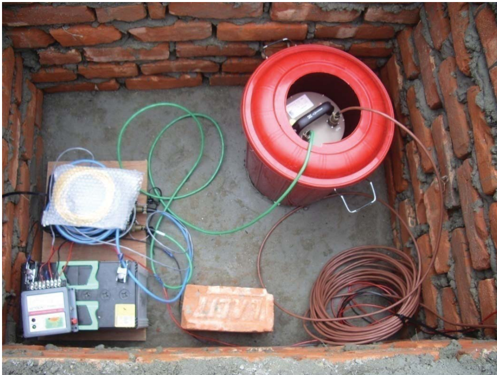
Fig. 15. Seismometer in the vault.
